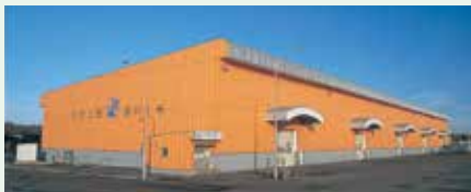
公共上屋樽川1号 ●5,000m 2 ・5t吊 天井 クレーン付 Tarukawa Public Transit Shed No.1 5,000 m 2 with 5-t roof crane
