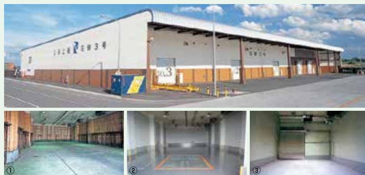
公共上屋花畔3号 ●4,000m 2 ・11.5mの底・3t吊天井クレーン付 Bannaguro Public Shed No. 3 4,000 m 2 in area, with 11.5-m-long eaves and a 3-ton roof crane 上屋に、くん蒸庫・定温庫を完備 The shed is complete with fumigating and thermostatic chambers.
